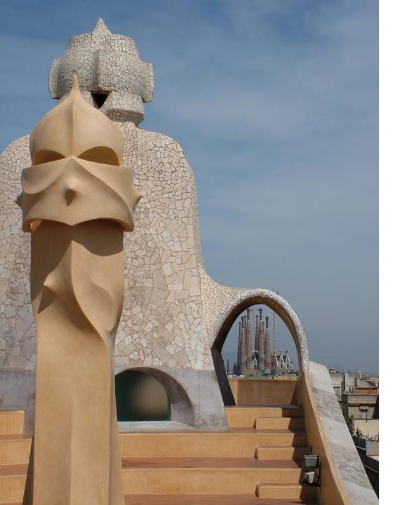
Note the twist in the stems. This helps the wind pass the chimney pot without damaging the surfaces.
